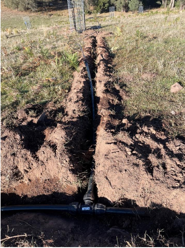
A large 1¼" poly pipe leads to smaller 19mm then 13mm pipes before terminating with a tap for each tree
