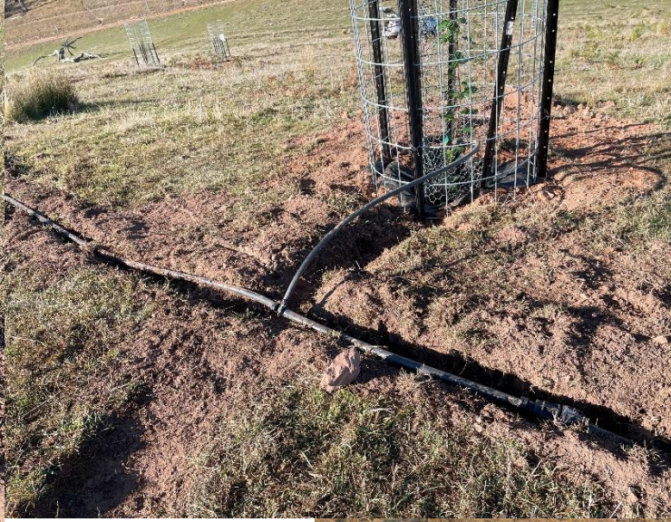
A large 1¼" poly pipe leads to smaller 19mm then 13mm pipes before terminating with a tap for each tree
